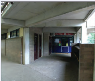
Figure 3 Former library entrance
