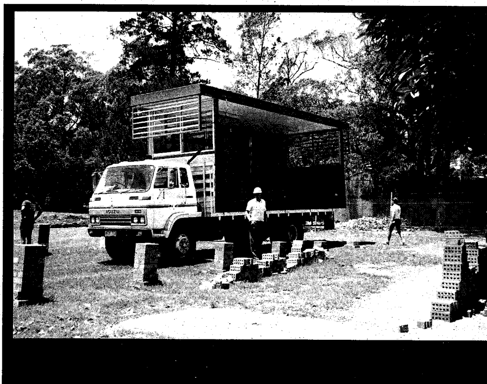
Demountable library arrives Feb 1988; remains of original library is in the background.
