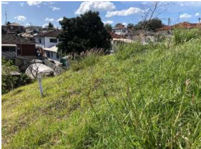
Picture 3 – Slope within north-western hotspot area
